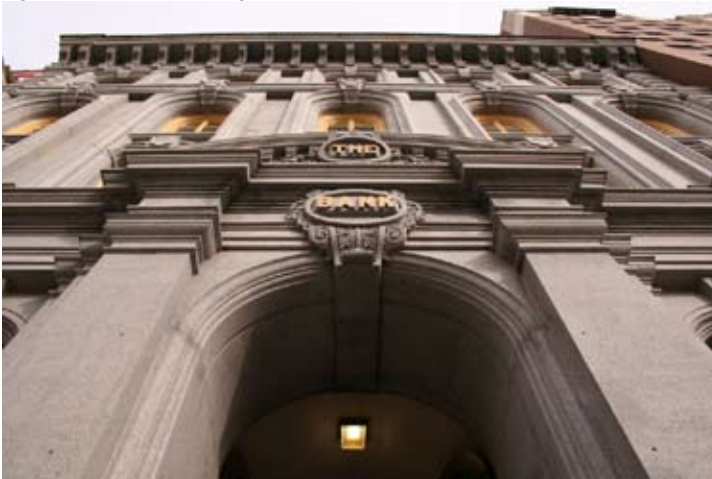
Figure 2 The Bank Building
